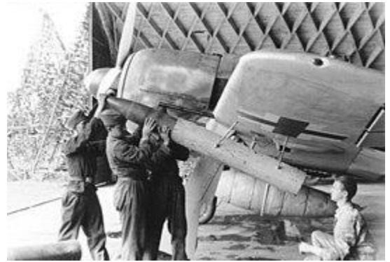
Fw 190A-8 with the under-wing WGr 21 rocket-propelled mortar. The weapon was developed from the 21 cm Nebelwerfer 42 infantry weapon.
