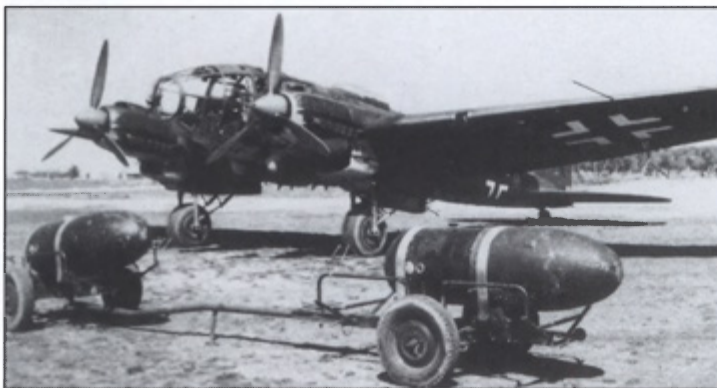
A pair of 500 kg LMAs (Luftminen 'A' or Aerial Mines Type 'A') wait to be loaded aboard a night-camouflaged He 111H
