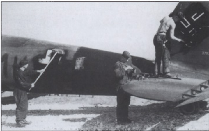
Most machines were soon being given a coat of washable black distemper as night camouflage
