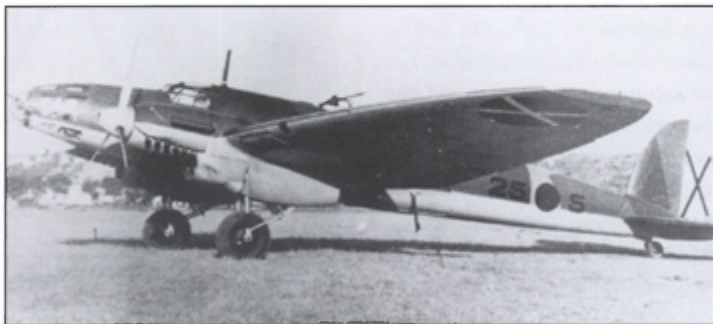
The first machine of the second batch of He 111B-1s to be sent to Spain, '25.5' would originally have been wearing an overall grey scheme upon its arrival in July 1937. By the time this photograph was taken it had been repainted in splinter camouflage to match later deliveries
