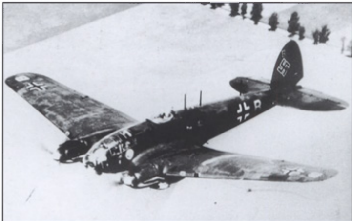
'6N+BH' was a typical KGr.100 'Dreimaster' ('Three master') pathfinder of the early war years. In this photograph the rearmost mast – mounted directly above the fuselage cross – is, unfortunately, difficult to make out against the starboard tailplane
