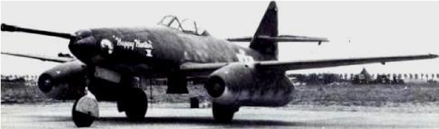
Messerschmitt Me 262A-1a/U4 Schwalbe, (Wk. Nr. 170083), "V083", "Pulkzerstörer", armed with one 50-mm Mauser Mk. 214 cannon. USAAF "Feudin 54" A.D Sq was painted on the port side of the nose of all the refurbished Me 262s, later painted over before leaving Lager Lechfeld Flugplatz and being shipped to the USA on HMS Reaper . This aircraft became Watson's Whizzers No. 000, with the name " Wilma Jeanne " on the starboard side of the nose, later the " Happy Hunter II ". This aircraft crashed on a flight from Lechfield, Germany to Cherbourg. (USAAF Photo)
